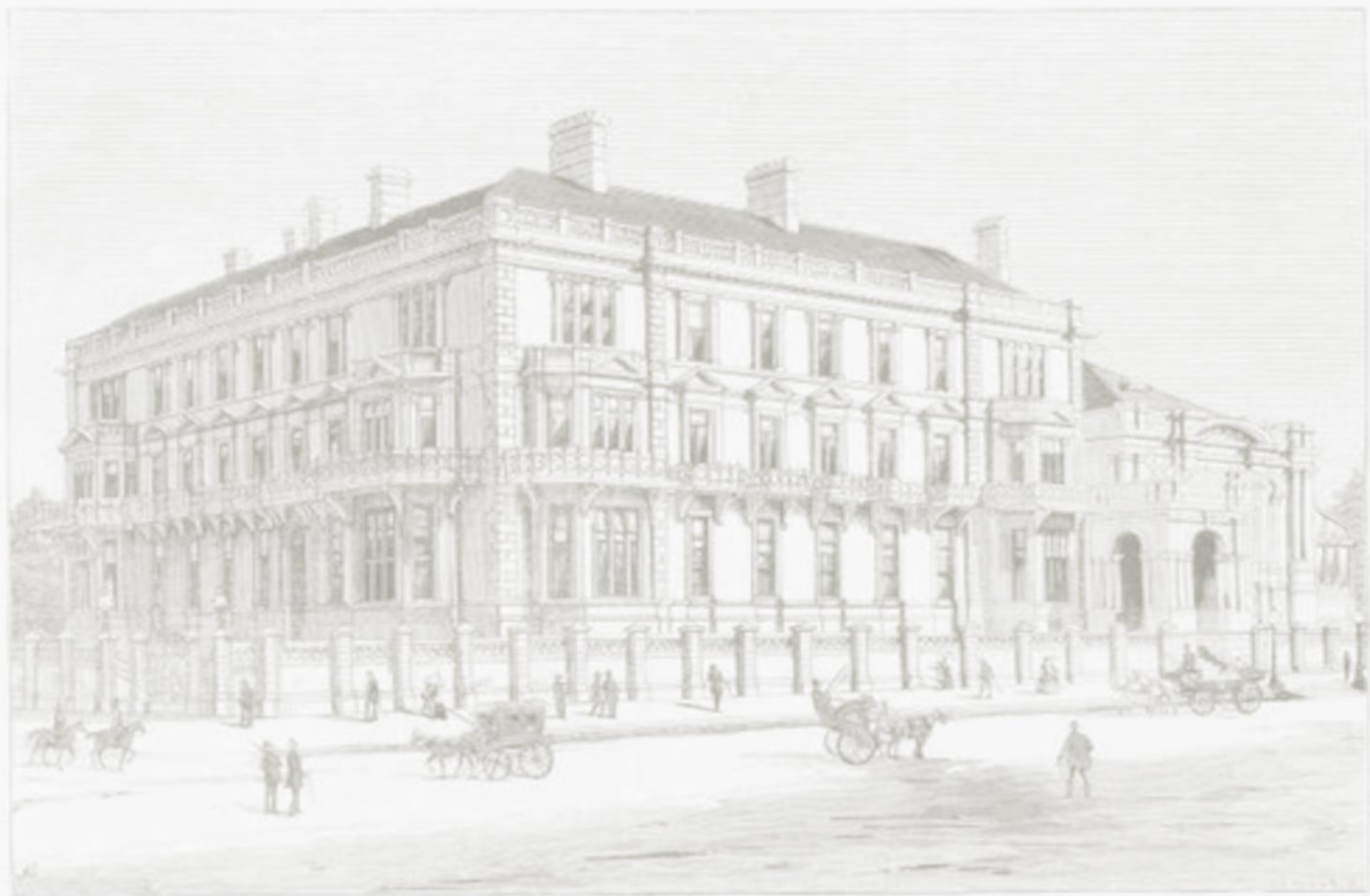
SIR W. J. CLARKE'S NEW RESIDENCE, EAST MELBOURNE
